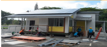
UTM Solar Home under construction
