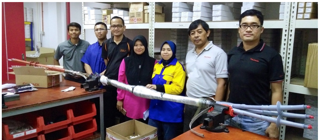
The completed PILC-XLPE transition cable joint.
