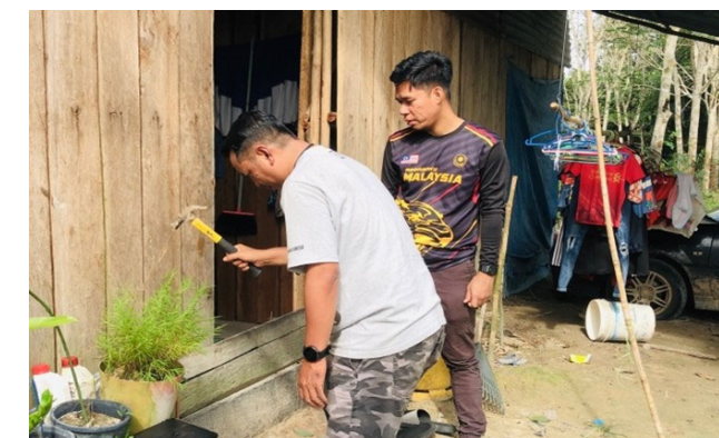
Relocation the solar system and solar panel
