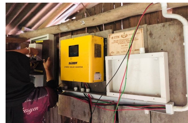
Dismantling of the solar system and solar panel
