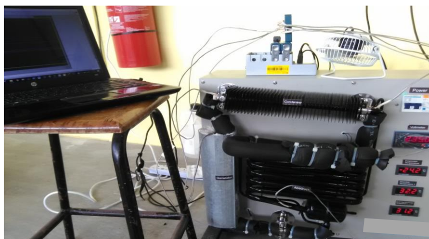
Absorption Chiller Operating Data Logging to Computer through NI Logger
