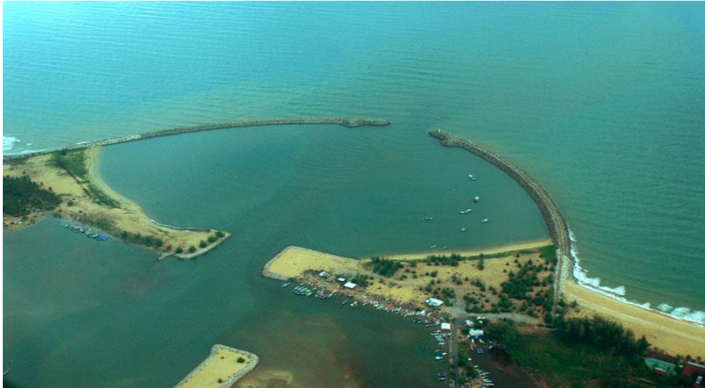
Figure 2.6 The aerial view of Kuala Terengganu breakwater
