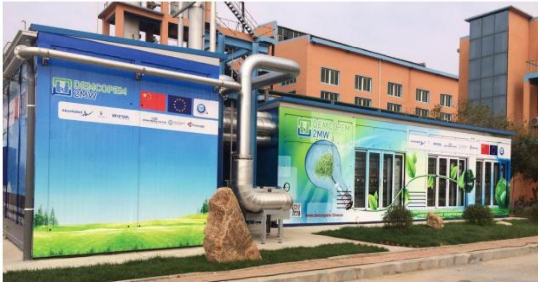
Figure 2.8 DEMCOPEM-2 PEMFC power plant at Ynnovate, Yingkou [58]
