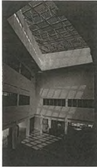
Atrium with glass semi-transparent PV modules (11.64kWp)
