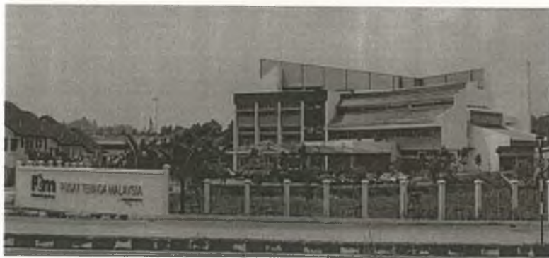
Colour of building exterior minimises heat gain
