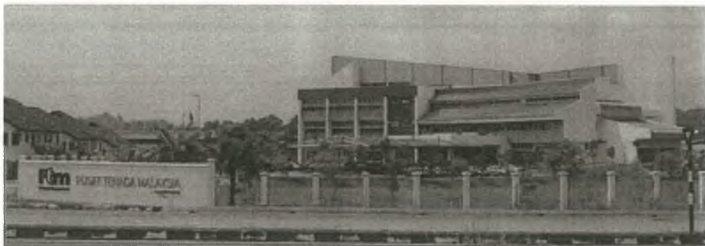
Colour of building exterior minimises heat gain
