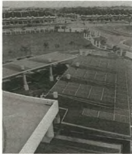
Monocrystalline PV modules (27kWp) on the car park roof
