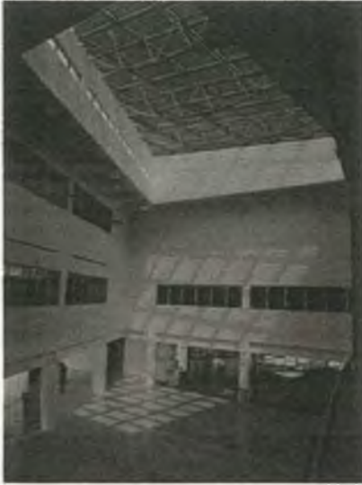
Atrium with glass semi-transparent PV modules (11.64kWp)
